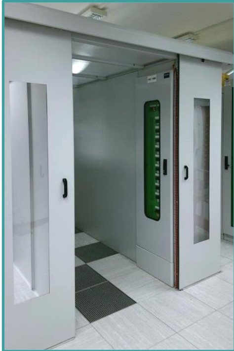
Fig. 1: Cold aisle containment
